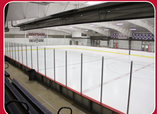
Energy efficient gas-fired radiant heaters improved comfort while saving energy
